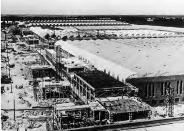
MAIN PLANT SHELL
