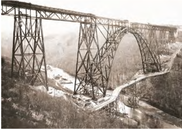
CONSTRUCTION OF THE MÜNGSTEN STEEL BRIDGE
