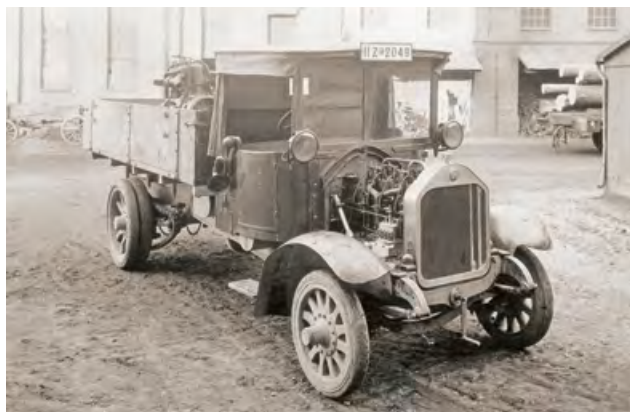
FIRST MAN TRUCK WITH A DIESEL ENGINE AND DIRECT FUEL INJECTION
