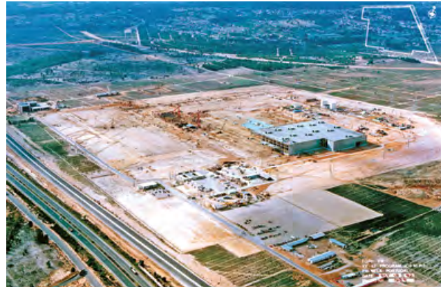
PALMELA PLANT SHELL CONSTRUCTION
